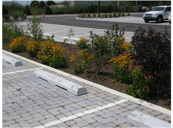
Parking - Permeable pavers and green infrastructure in parking area.
