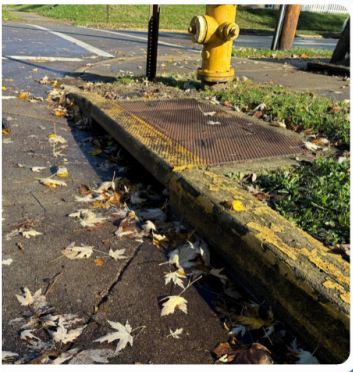
BEFORE with debris blocking drain
