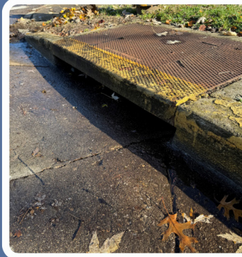
BEFORE with debris blocking drain
