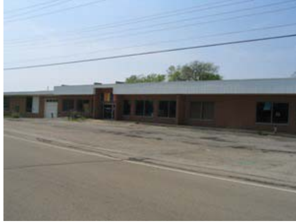
Photo Caption: The former Boathouse property on Marina Drive is scheduled for demolition on May 17.
