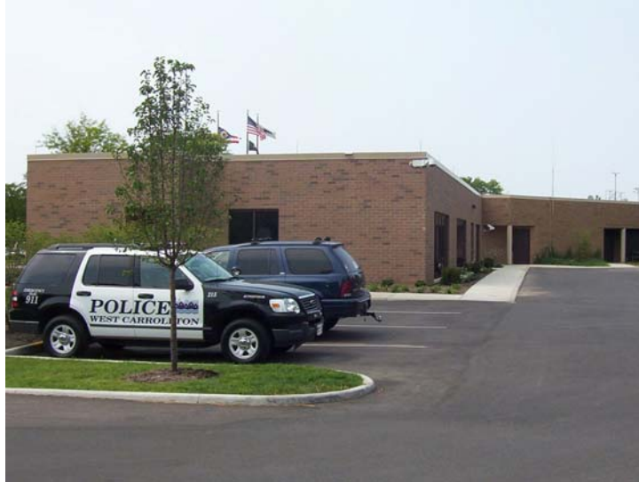
The West Carrollton police department addition to the Civic Center was recently completed.
